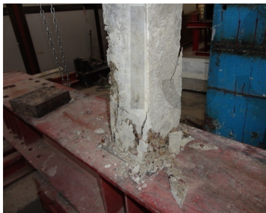
Figure (4) Failure pattern of control column
